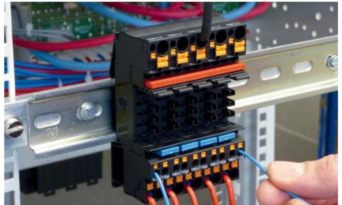
**5** Push in the two cables for the series connection of the auxiliary contacts
