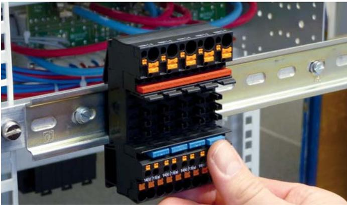
**2** Push in jumpers for group supply (here: series connection of auxiliary contacts)
